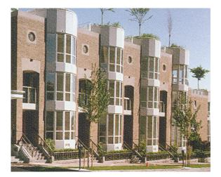
Vertically modulate the building using repeating patterns of bays, exterior stairs, railings, and recessed entries that express individual units.
