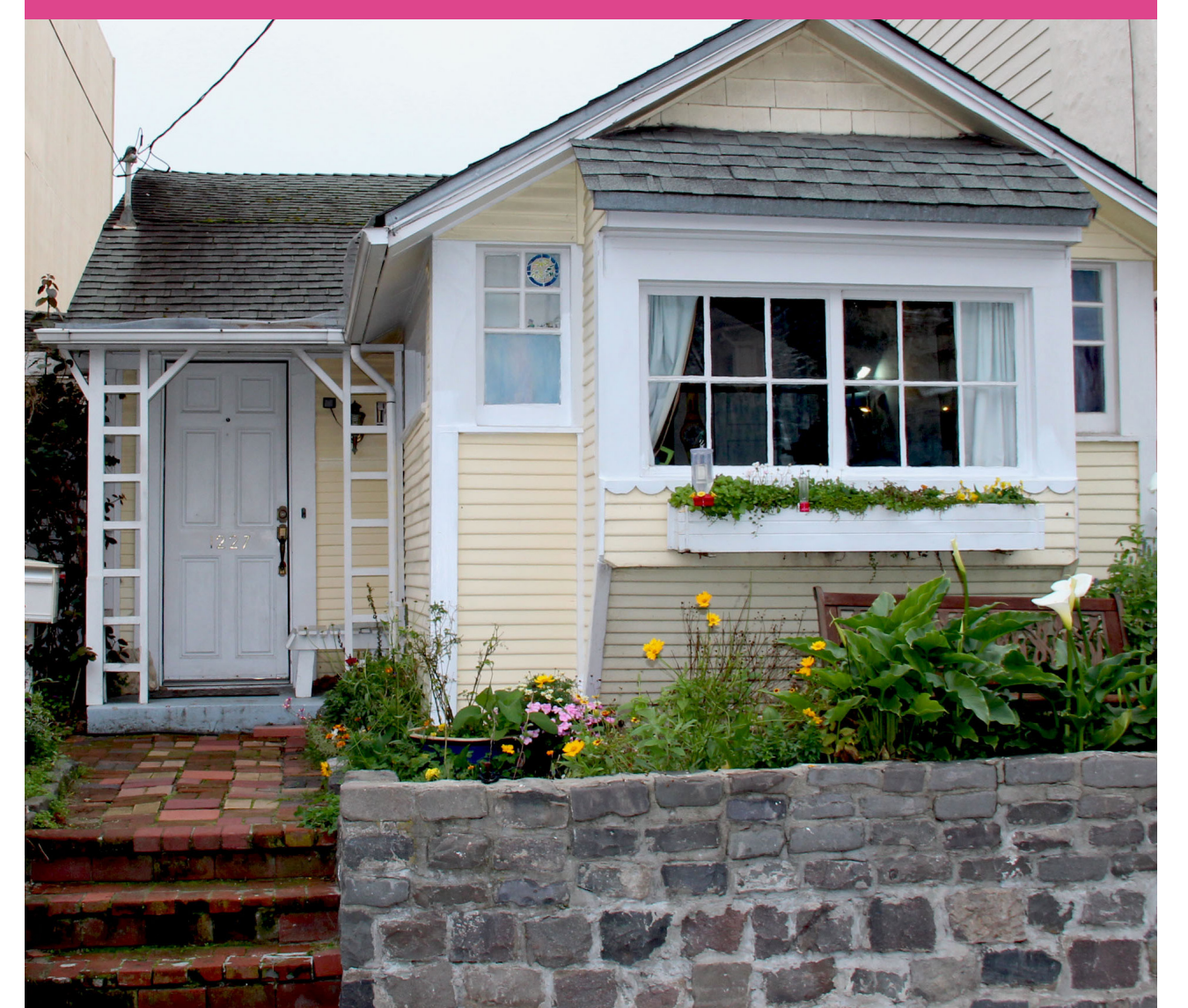
Earthquake Refugee Shack, Landmark No. 171
